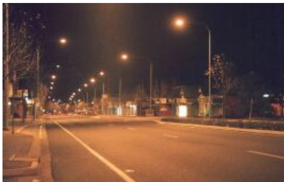
Quality full cut-off road lights on Sir Donald Bradman Drive reduce glare and facilitate night vision
