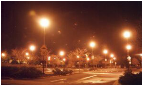
Glary globe-lights at a car park waste light sideways and upwards and contribute to skyglow
