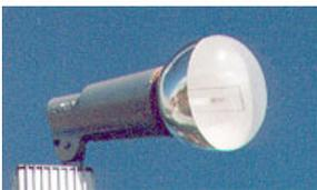
**BAD** No consideration was given to aiming nor shielding this floodlight. It is excessively glary and half of the light shines wastefully skyward!
